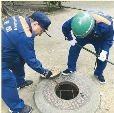
▲防火貯水槽の点検
